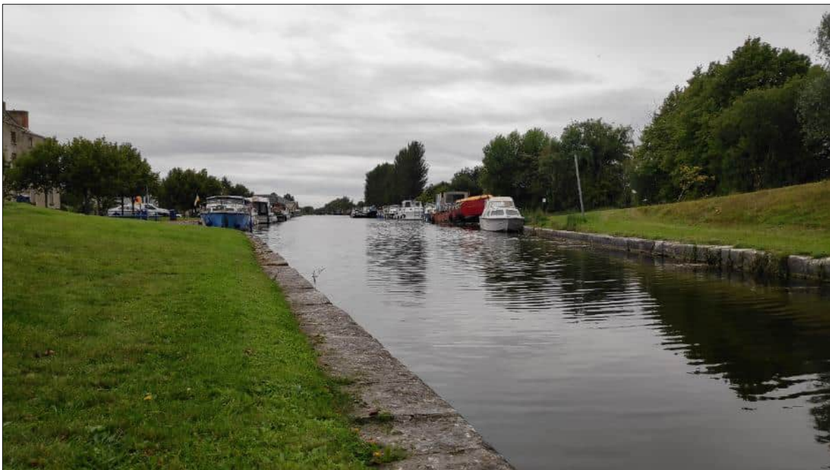
Plate 4.23 Representative image of site D4 on the Grand Canal at Griffith Bridge, August 2022 (facing westwards from bridge)
